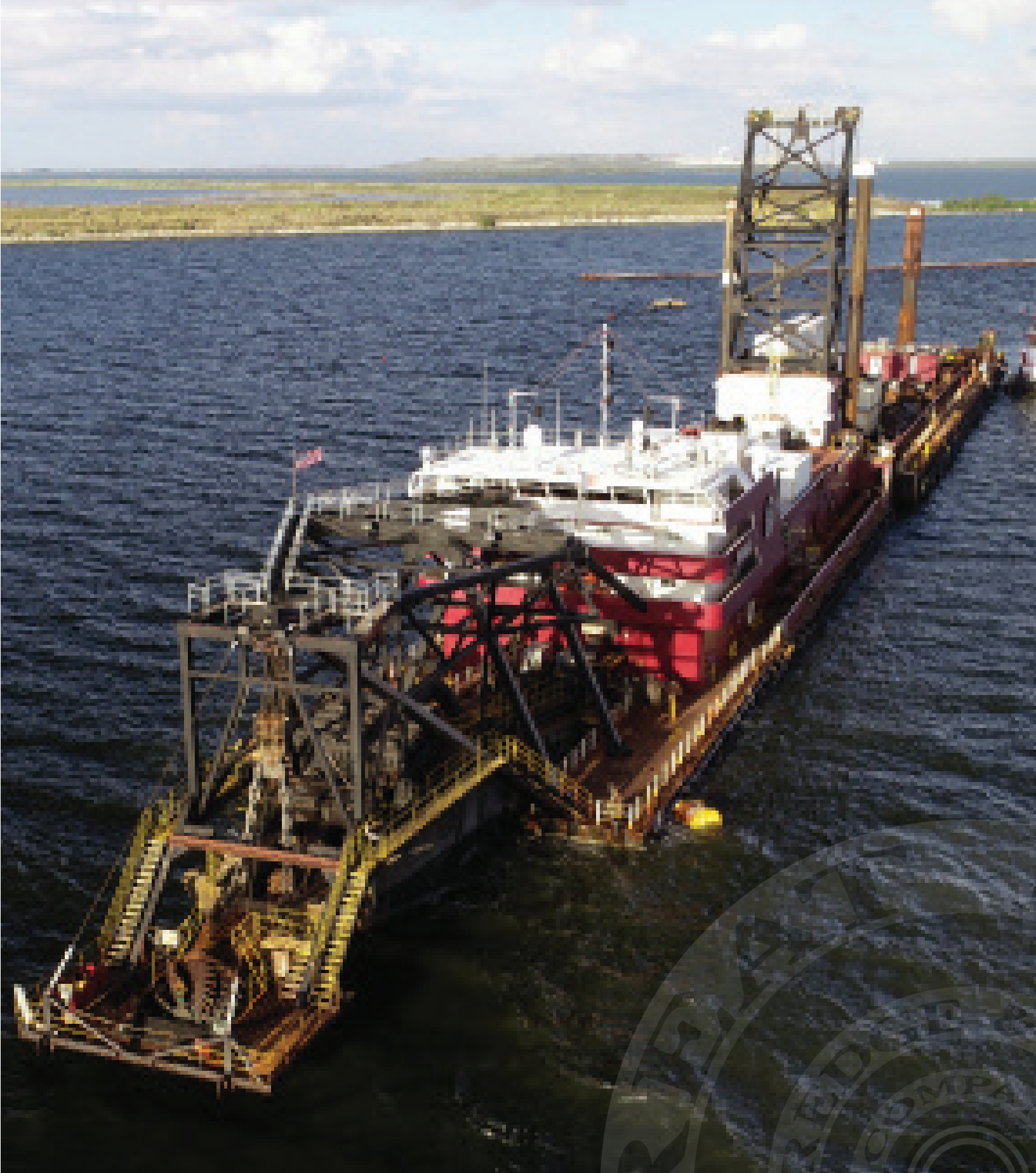
Photo: The Dredge Carolina mobilizes to the Corpus Christi Entrance Channel.
