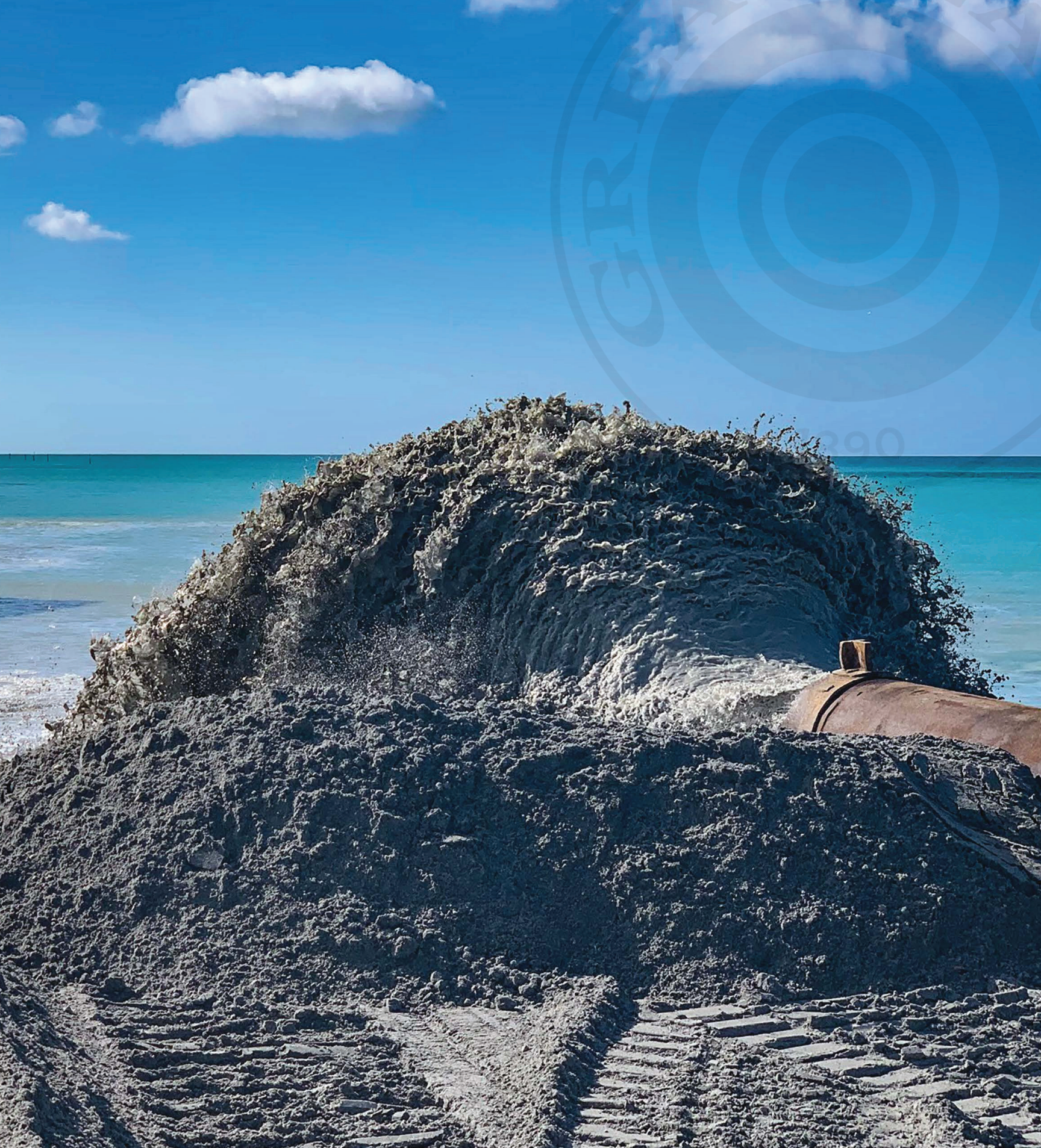
Beach pump out at Charlotte County, FL.
