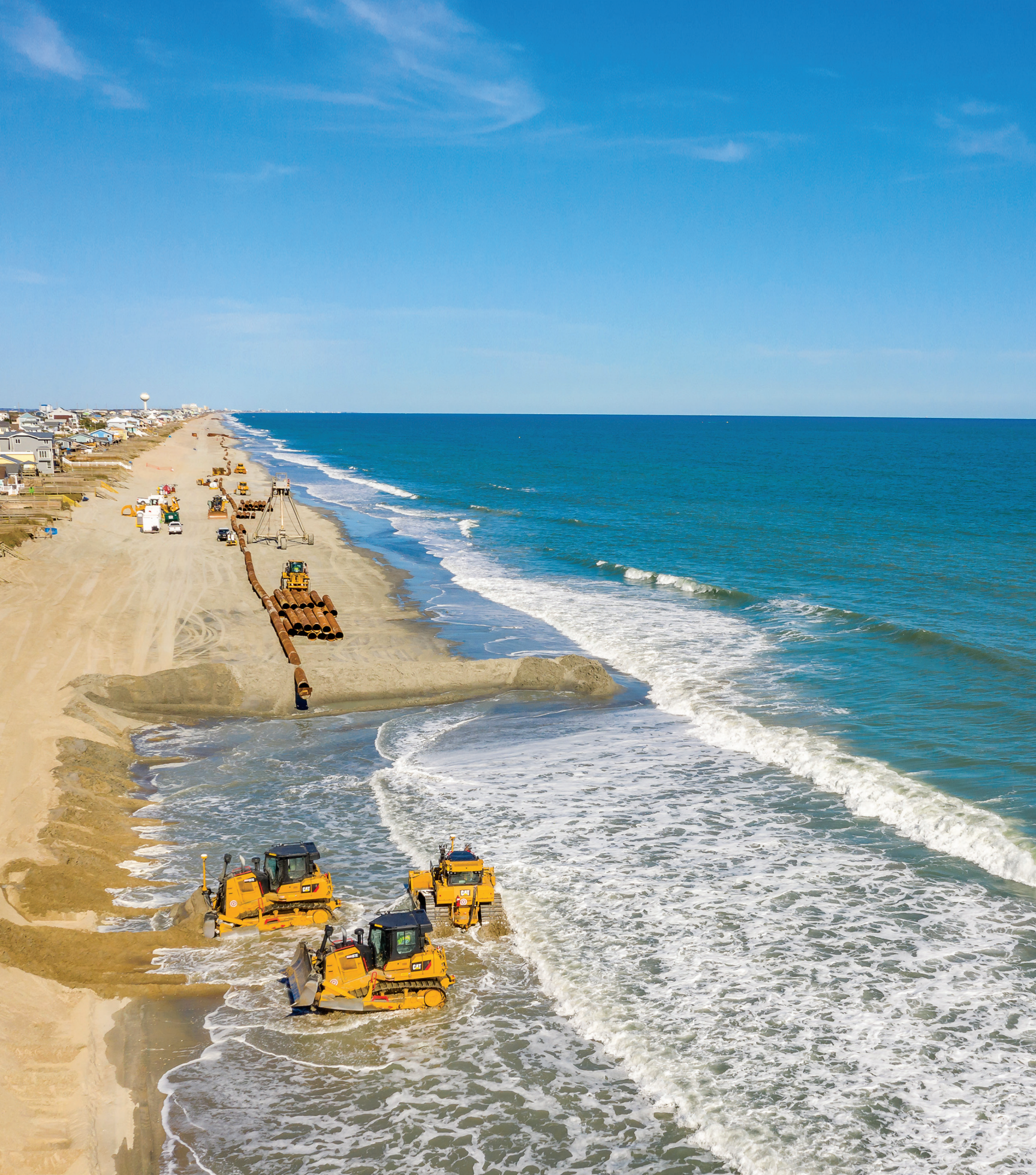
The Dredge Ellis Island offshore (far right) pumping to the beach. Emerald Isle, NC, Beach Nourishment Project. Photo: Brad Styron
