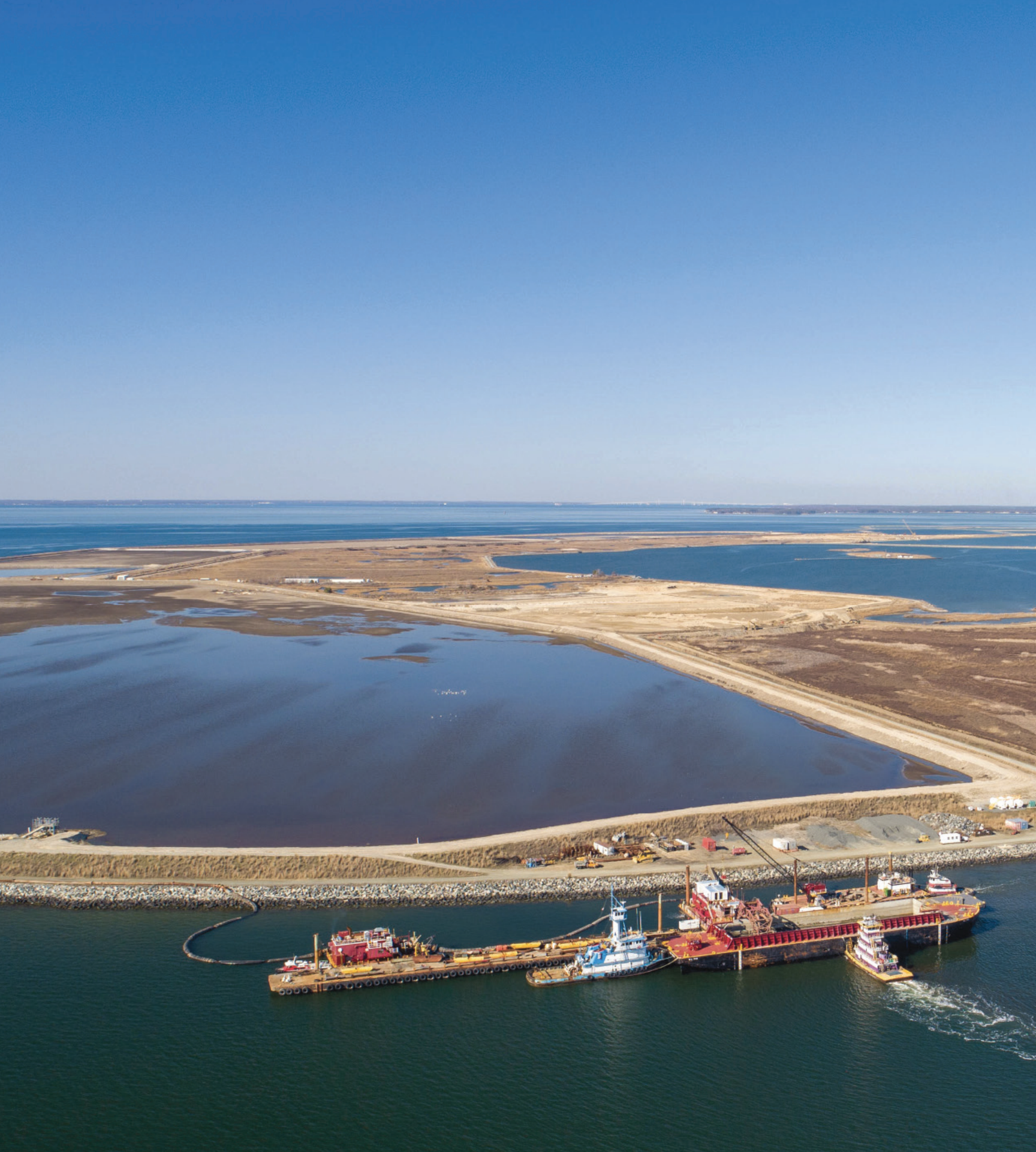
Unloader #2 at Poplar Island, Chesapeake Bay, MD.
